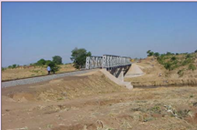
View of Lupanga Railway Bridge
