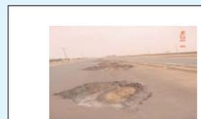
Photo 5: Pavement Premature Failure
