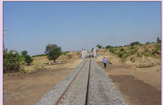
View of Lupanga Railway Bridge
